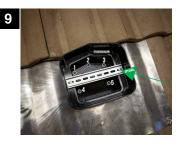
Secure the JB-2 to the roof decking using (5) #10 x 1-1/4" Phillips pan head screws (provided). Install outdoor-rated, UL 514B, NEMA 3R approved fittings and/or strain reliefs to the EAST, WEST and SOUTH side walls of JB-2 and complete wiring installation. Up to 1" raintight fittings are all acceptable. Clean off all burs.
