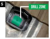
Place the JB-2 base into the opening in the flashing. Using a drill bit, drill through the box & roof simultaneously within the approved 'Drill Zone'. Verify penetration hole(s) are on either side of a rafter but not over or through a rafter/truss.
