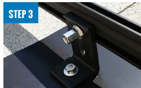
ATTACH L-FOOT TO RAIL
