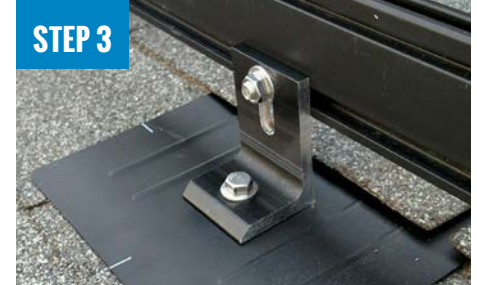
ATTACH L-FOOT TO RAIL
