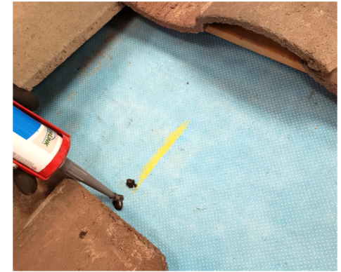
4. Remove hook, clean debris and fill pilot holes with roofing sealant
