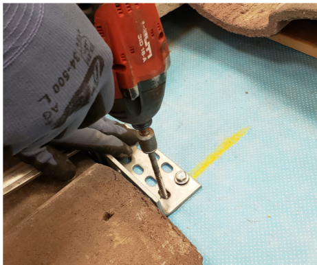
5. Reposition hook, secure with included lag screws.
