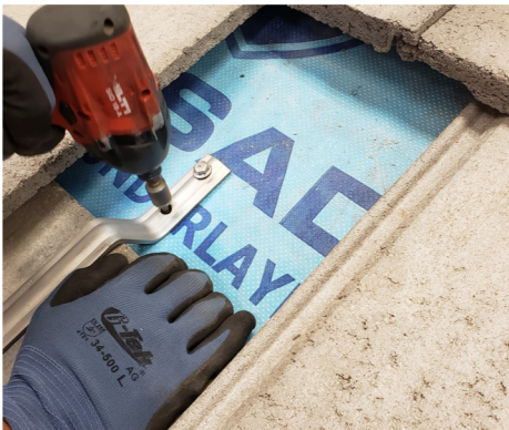
5. Reposition hook, secure with included lag screws.
