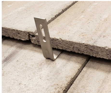
6. Replace tiles, if necessary notch with grinder to ensure proper fit.
