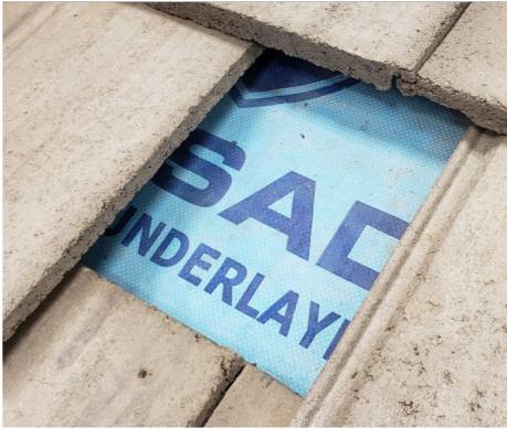
1. Remove tiles around installation area.
