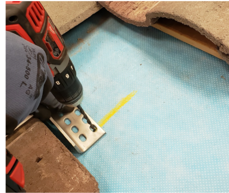
3. Position hook, adjusting arm-base bolt position as needed. Use 3/16" bit to drill 2 pilot holes.
