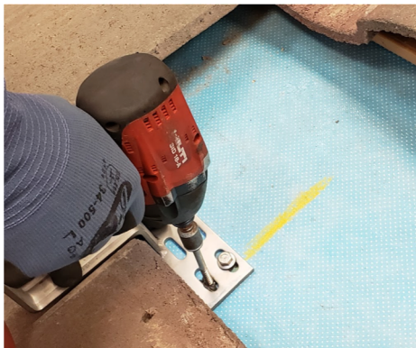
5. Reposition hook, secure with included lag screws.
