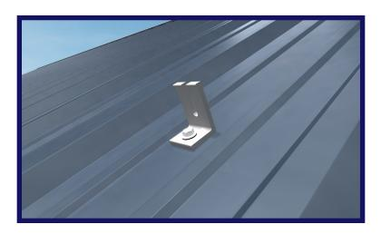
Tighten fastener until bracket is pulled down snug to the roof surface. The tension required will vary with the project roof deck, age, and type. Be sure not to over tighten the fasteners and strip the threads.
