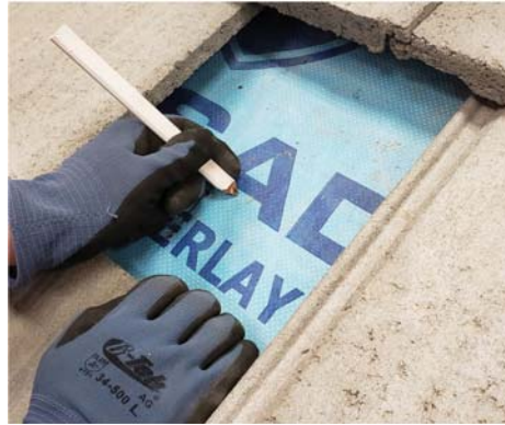
2. Locate and mark rafters.
