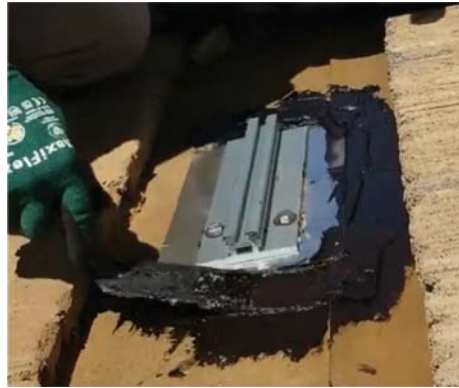
2. Using Margin Trowel, apply base coat of roofing cement.
