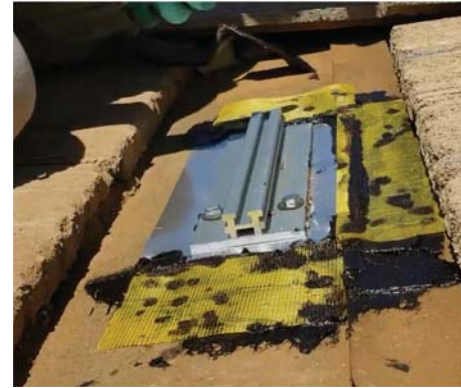
3. Cut roof repair fabric size, lay into roofing cement.
