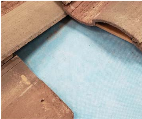
1. Remove tiles around installation area.
