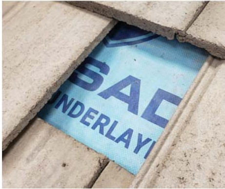
1. Remove tiles around installation area.
