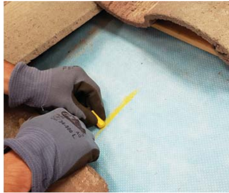
2. Locate and mark rafters.
