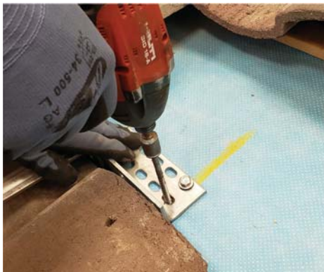
5. Reposition hook, secure with included lag screws.
