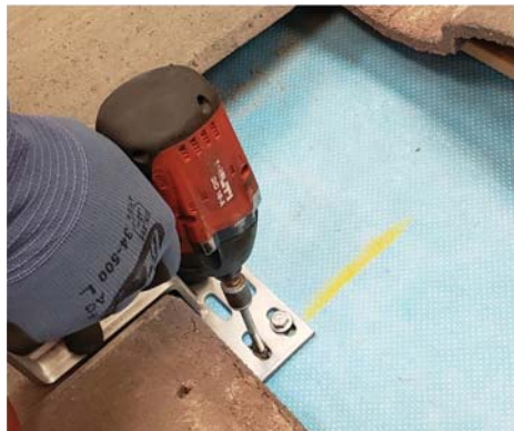
5. Reposition hook, secure with included lag screws.
