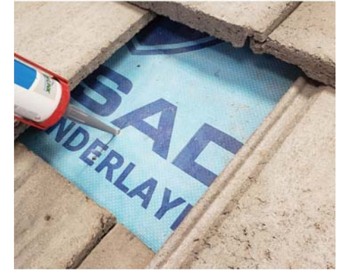
4. Remove hook, clean debris, then fill pilot holes and rib on back of hook with roofing sealant.
