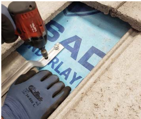
5. Reposition hook, secure with included lag screws.
