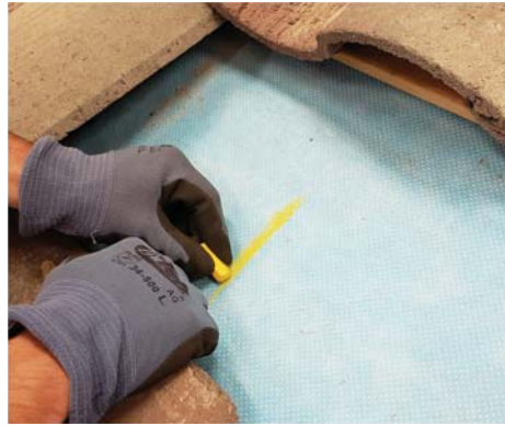
2. Locate and mark rafters.
