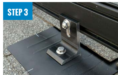
STEP 3 ATTACH L-FOOT TO RAIL
