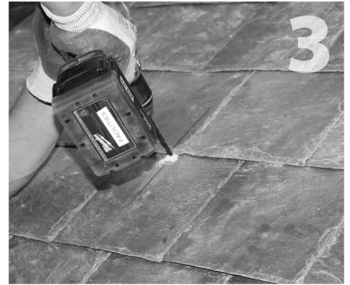
Using a masonry drill bit, drill a pilot hole at the center of the QBase location you marked in step 2. This drill bit should match the size of the guide bit of your hole saw.
